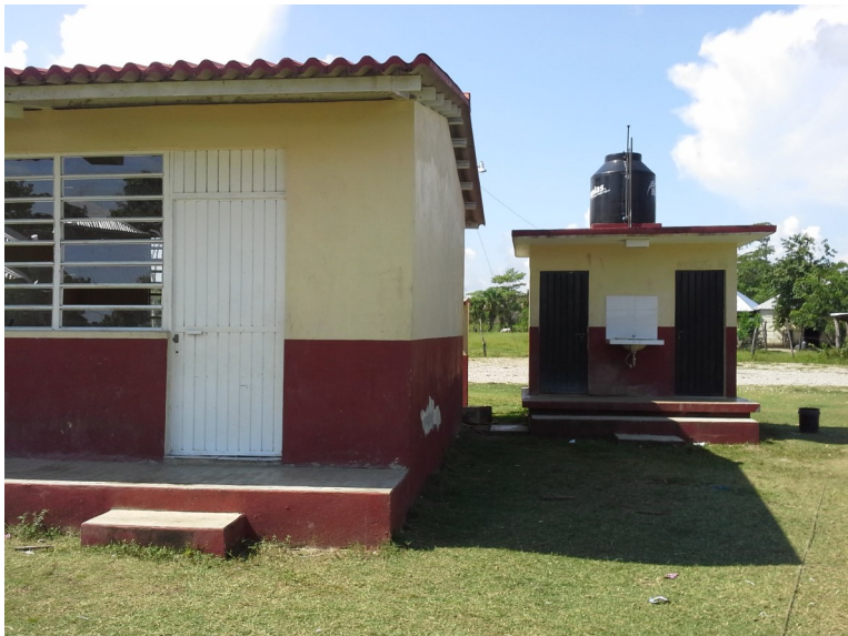
Schoolhouse classroom and bathroom structures in El Piñal, Tabasco, are elevated to avoid inundation from flood water. The black tank on top of the bathroom provides water and pressure to maintain sewage disposal. The facility can serve as a safe meeting point and provide clean water for the community during floods.
