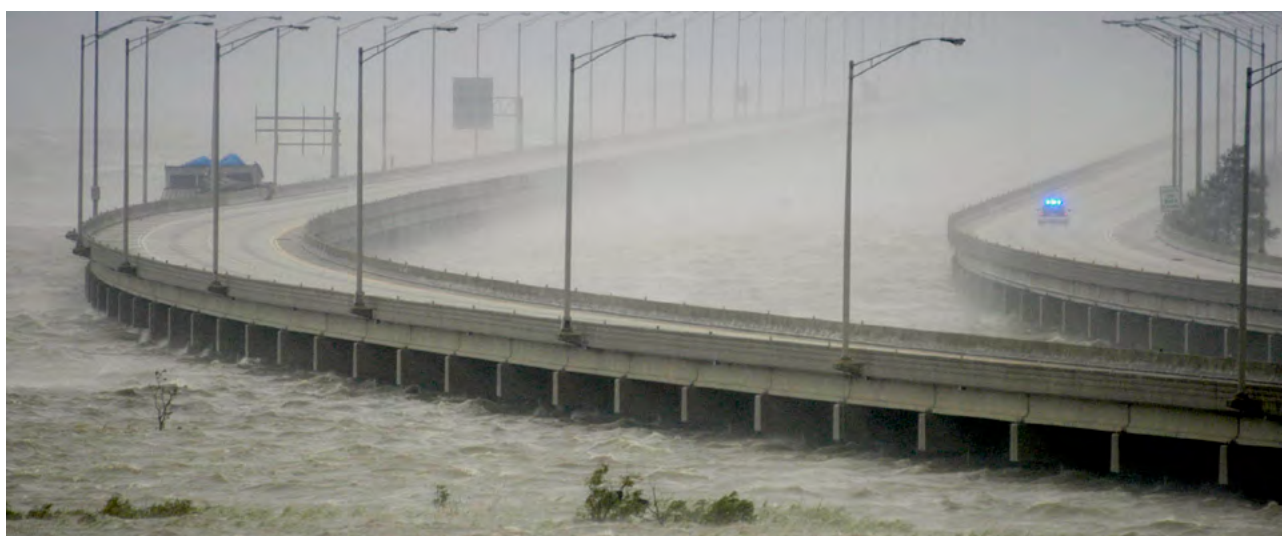
Flooding caused by Hurricane Katrina, 2005
